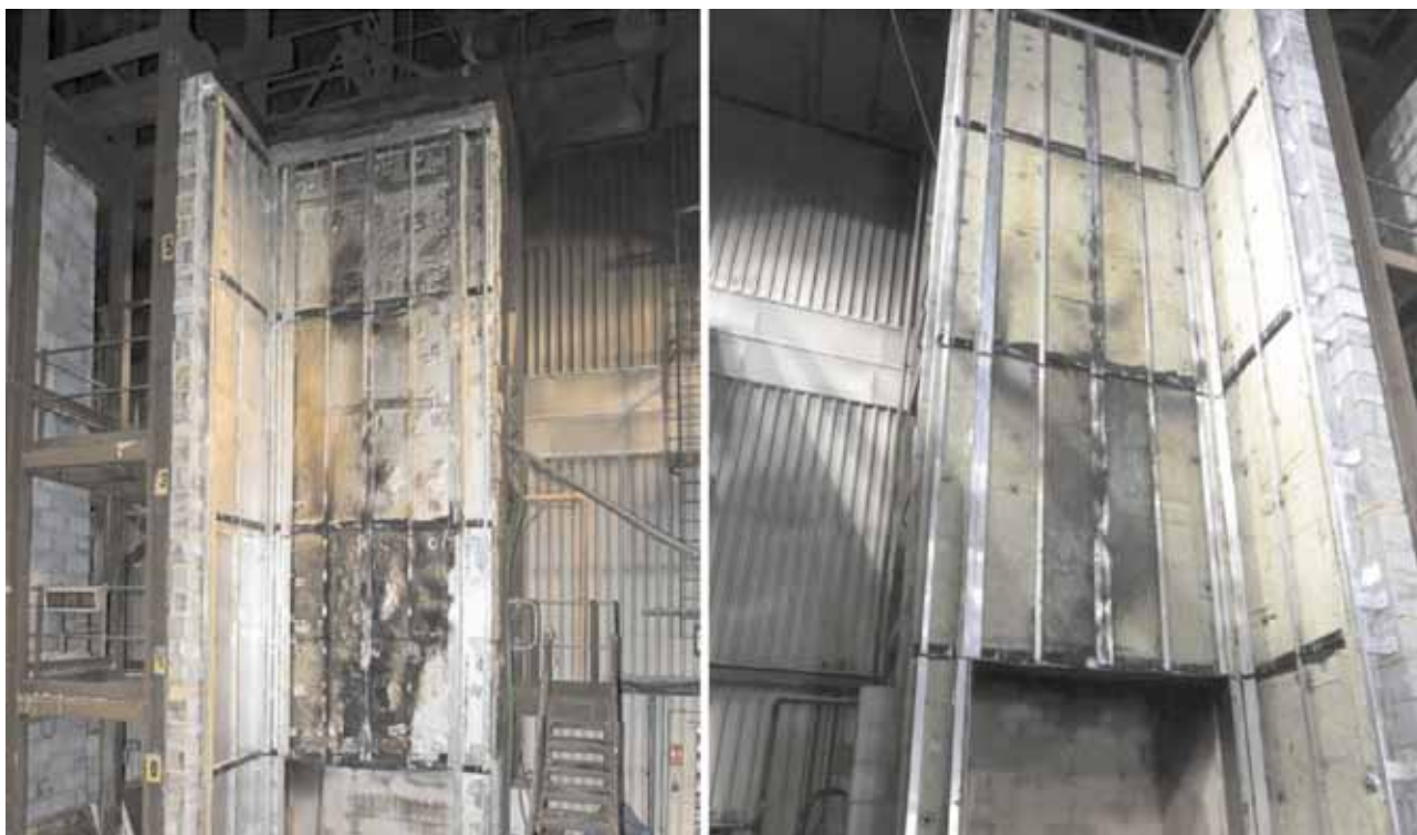
Fig. 4. The PIR (left) and stone wool insulations (right) after BS8414 tests no. 1 and no. 2 and removing the ACM (PE) decorative cladding
